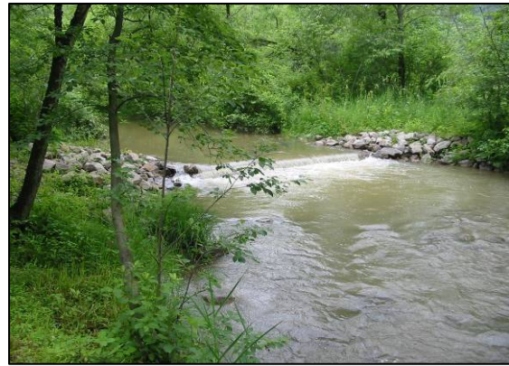
Fish habitat improvement project on Cherry Run
