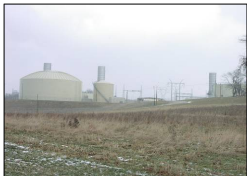
Dominion Armstrong Energy, LLC Power Station gas fueled power plant in South Bend Township
