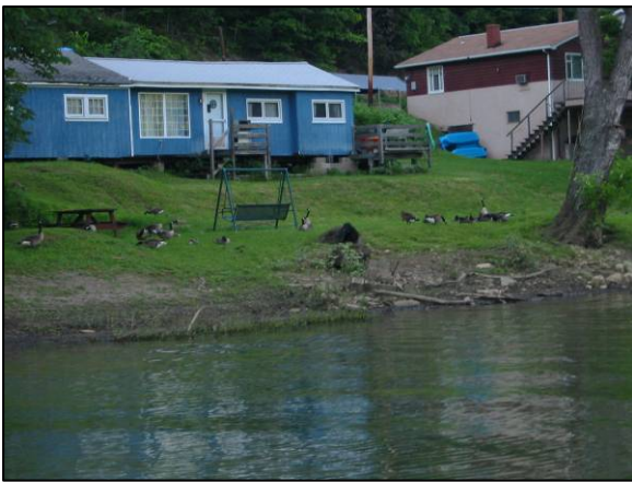
There are many old 'camps' along Crooked Creek with inadequate septic systems
